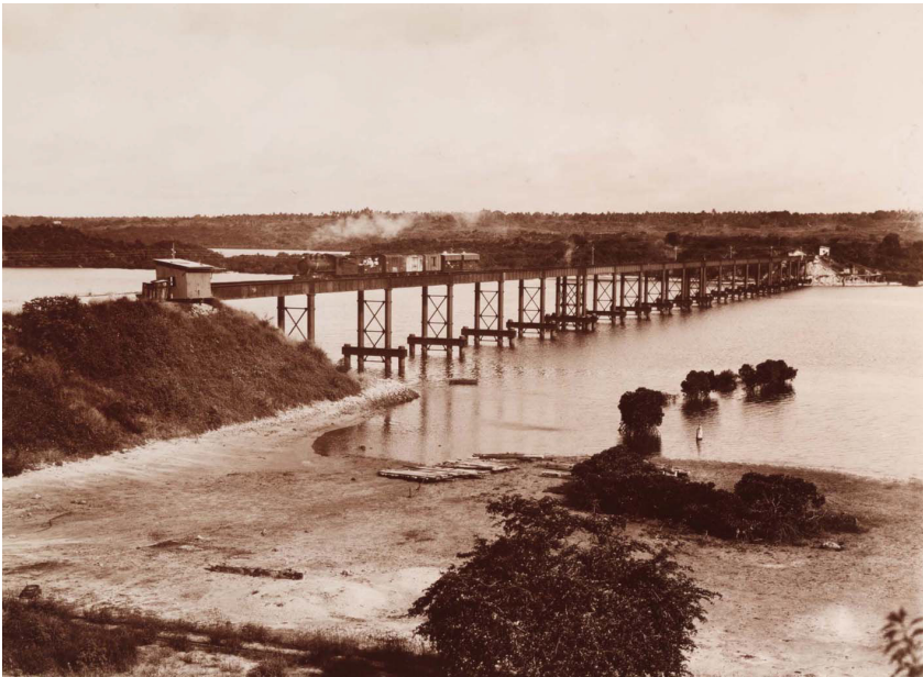
The Salisbury Bridge, Mombasa 1899-1901
