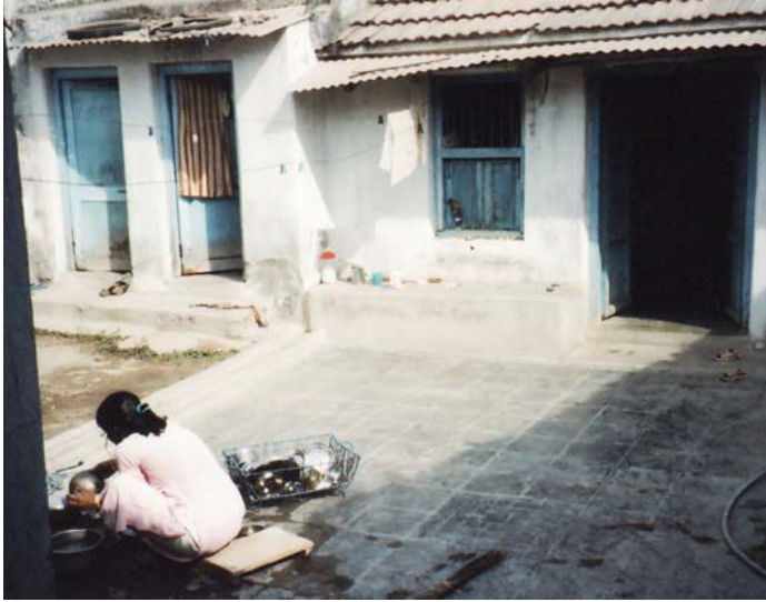
Padana dwelling: Open court yard, No 4 on plan (door to No 5 and 8 in background)
